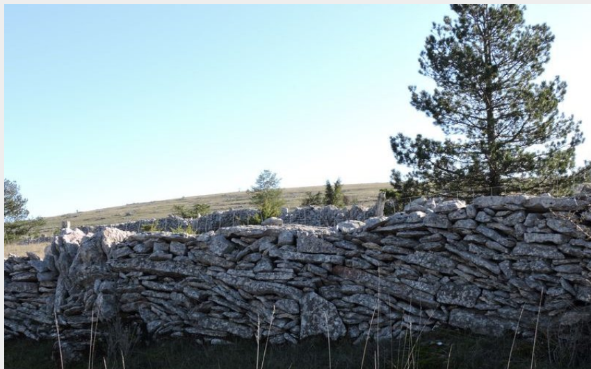
Murets (© OTGCC nc)
